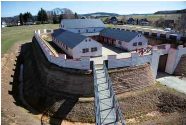
Earth wall from the earliest Limes period, made of stacked turf blocks, and timber-framed buildings with painted facing panels imitating ashlar masonry.
