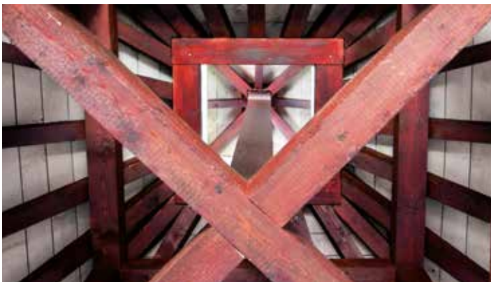
Replica of a watchtower at Pohl. View of the roof structure with radial rafters, open lantern for channelling smoke and sturdy shaft for the wooden pinecone crest.
